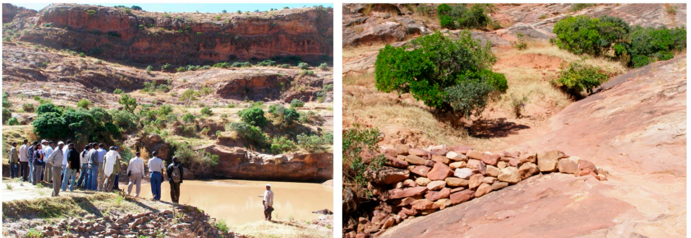
Figure 6. Catchment interventions. (left): small dam, (right): runoff-stopping structure. Tigray, Ethiopia [45].
