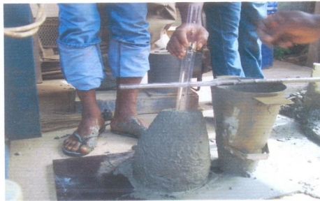
TEST OF WORKABILITY OF CONCRETE
