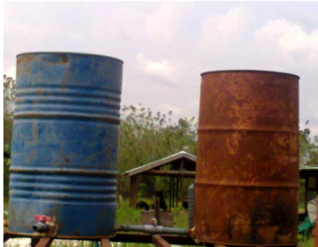
Plate 1. Storage tank serves as reservoir to supply water to the main pipeline
