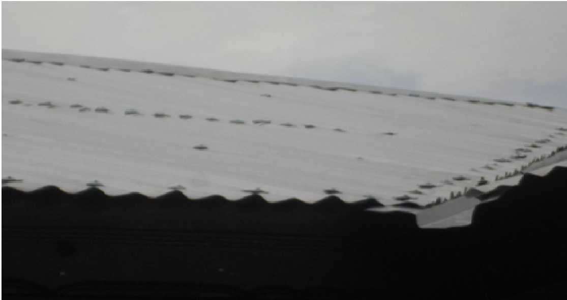
Plate 3. Aluminium roof where samples were collected
