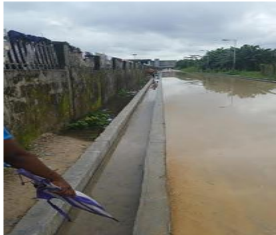
Plate 2. Dampness of walls
